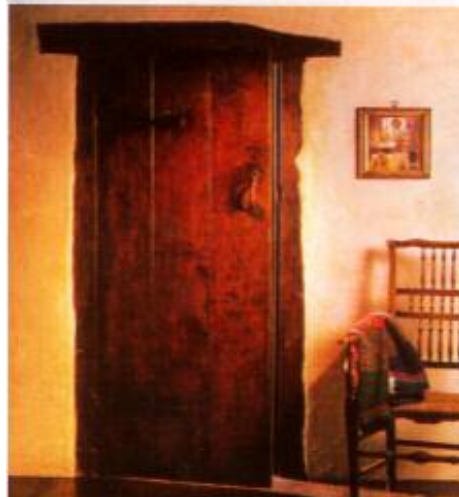
CW2 The Warnham Three plank door with beaded and rebated joints
