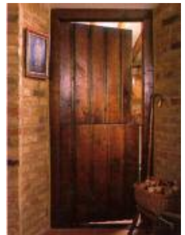
CW5 The Petworth (5 plank version) Five plank door with rebated joints and ogee mouldings
