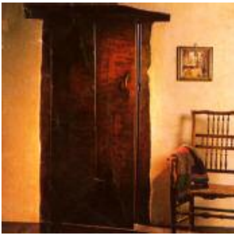
CW1 The Nutbourne Two or three plank door with angled butt joints
